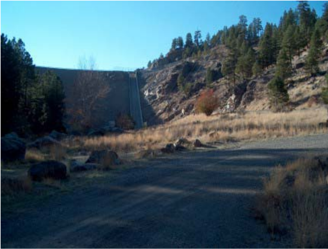
Figure C-8. Transmission line grassland (top) and parking lot grassland (below).
